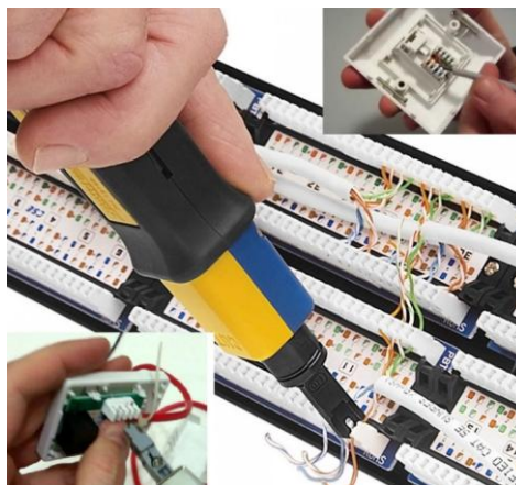
Rajah 3 : Cable termination
