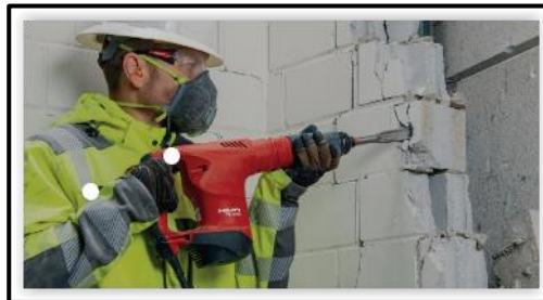
Rajah 15: Demolition Hammer
